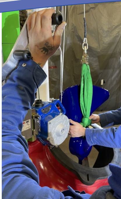
② 02 Davit lifting system used as a hoist for inserting a glass-lined stirrer into a stirrer vessel.
